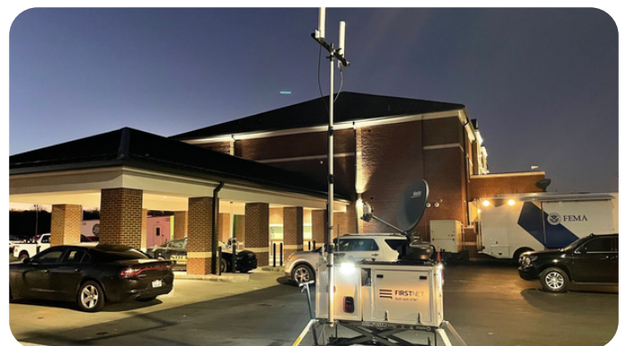
Hospital and FEMA Tornado Command Support
